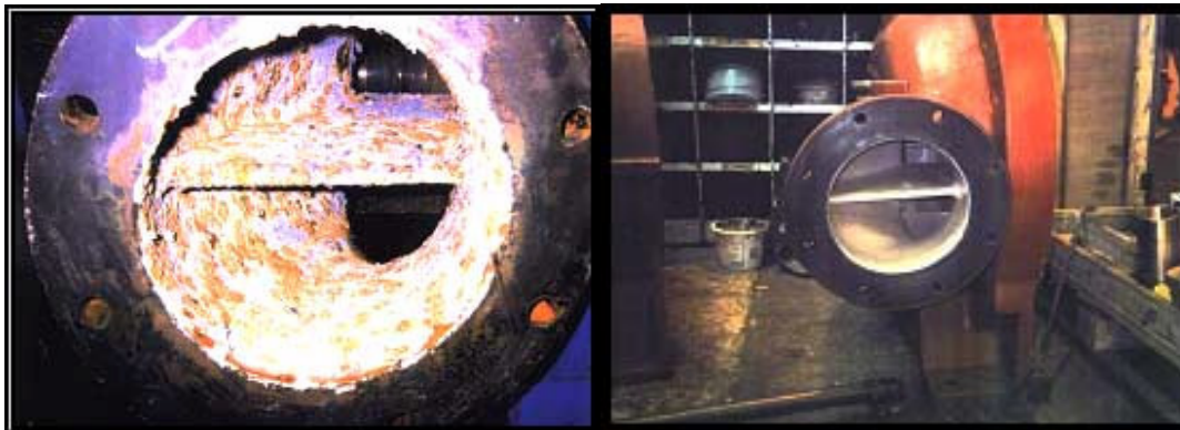
Figure 3-6 Worn pump inlet before and after repair and coating with low friction protective coating, (courtesy Corrocoat, Leeds, UK).
