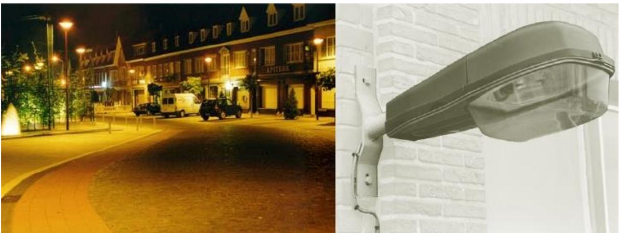
Figure 3-20: Street lighting luminaires attached to poles(left) and to a house (right)
