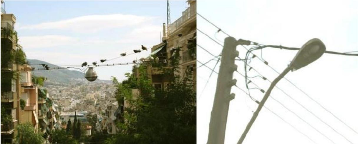
Figure 3-19: Street lighting luminaire attached to cables(left) and to electricity distribution (right)
